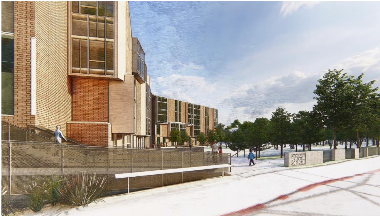
Park Entry from Westbourne Terrace
